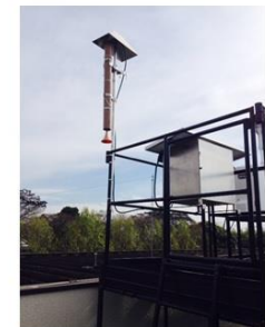
System installed at INPE's main campus
